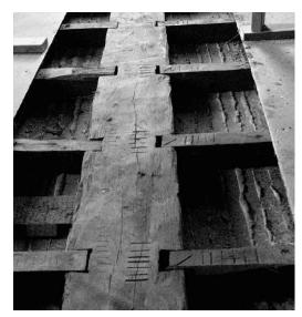
ioists and beams the became visible These pieces were hand-hewn on the ground and marked so that the correct joist went in its previously fitted slot. In this photo taken in the Master Bedroom, you can clearly see the sequence of chiseled markings in the wood. The other photo provides a close-up of two separate markings. It's interesting to see the methods that were used for
