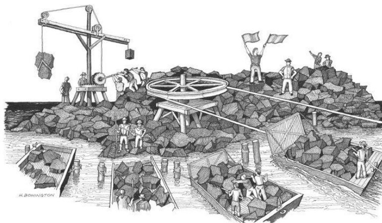
Construction of the West Dennis Breakwater by Howard Bonington
